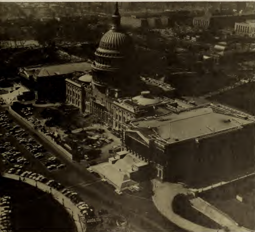
During the extension of the east front between 1958 and 1962, the original sandstone portico was removed. It was replicated in marble in front of the 32 feet of added space.
